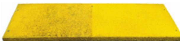
Example showing before and after high pressure cleaning
