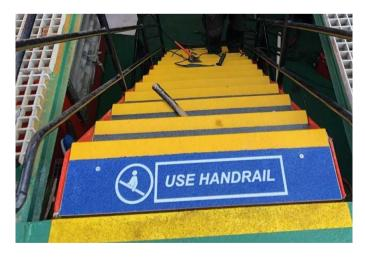
Figure 16: Real Safety anti-slip stair tread covers at Danish ship. Source: Author
