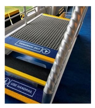
Figure 17: Formed KAG handrail sample. Source: (Appendix 1: Electronic Interviews).
